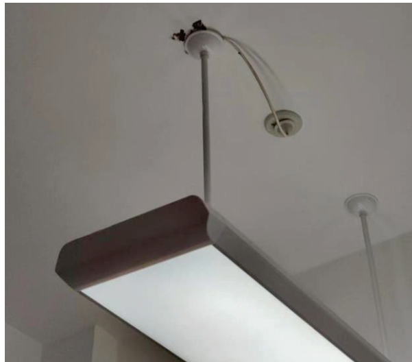
Figure 11. Classroom light with exposed power cord
