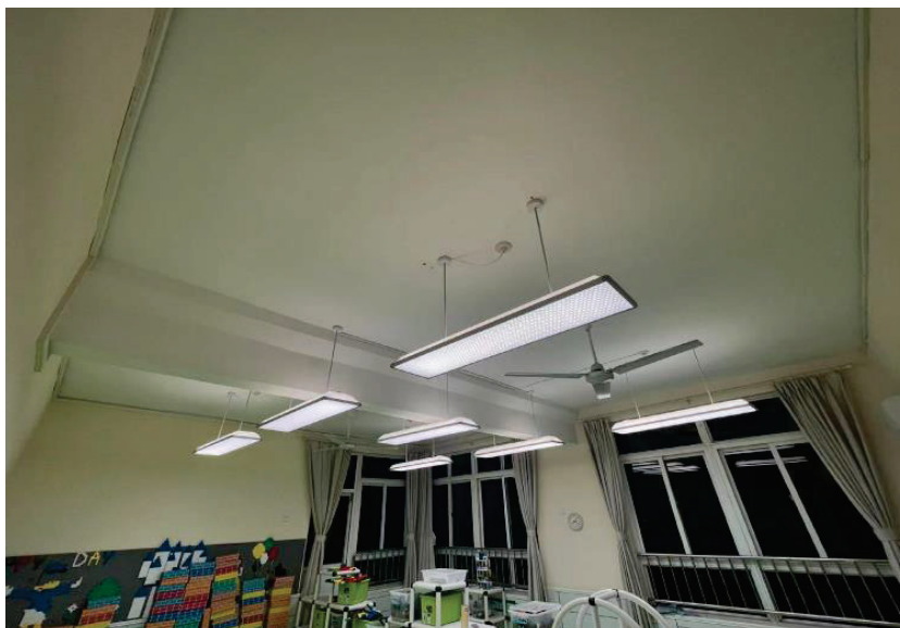
Figure 5. Classroom with overly concentrated lighting installation positions
