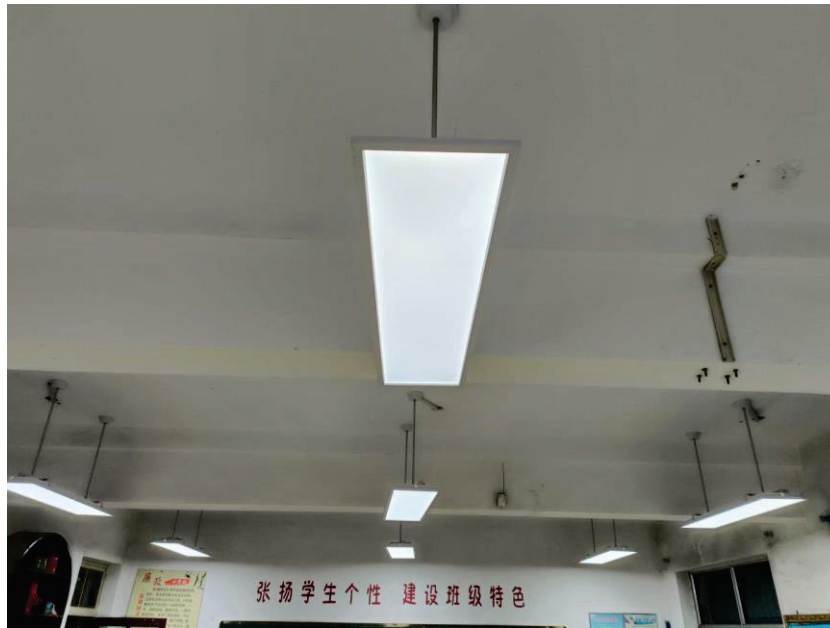
Figure 10. Classroom with Unneatly Installed Luminaires
